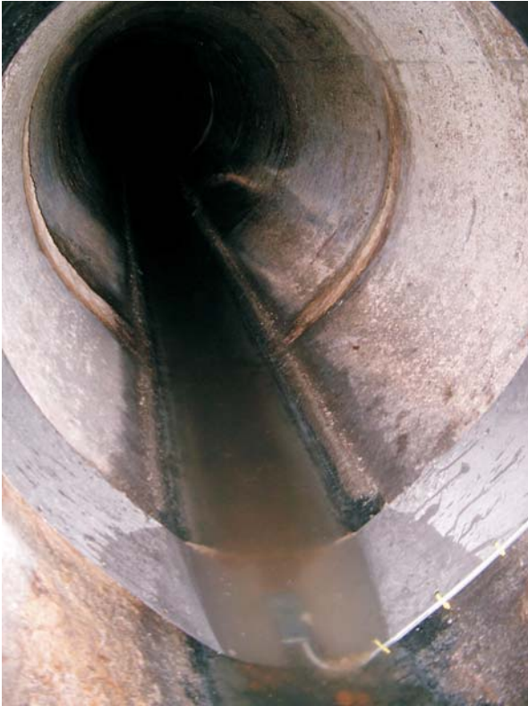
Sensor and Mounting Band installation in egg-shaped pipe
